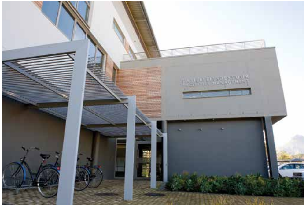
The modern and "green" Facilities Management Building is situated next to the Eerste River on the Stellenbosch Campus. Photo: WERNER ROUX
